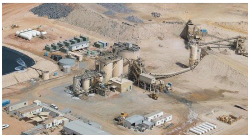
Figure 6 Central Gawler 650ktpa gold processing plant
