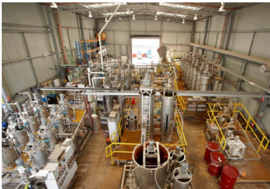
Figure 6 The CSIRO/Direct Nickel pilot plant in Perth WA
